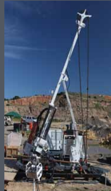
Surface Coring Rigs
